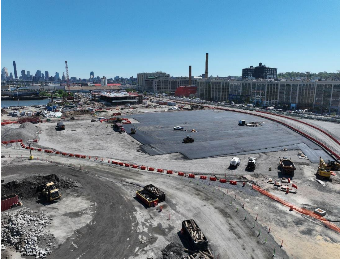
Port Staging Area – 05/19/2025
